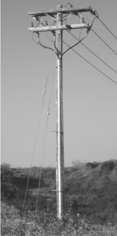
Figure 5-27 Dip pole or riser pole.
