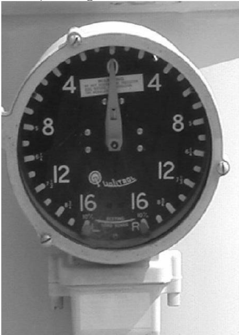
Figure 4-19 Regulator dial. Courtesy of Alliant Energy.
